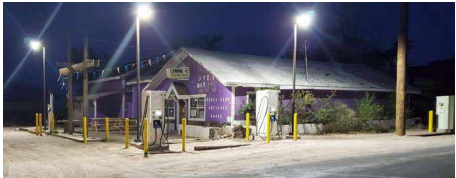
Photo (Above): NV Energy's NEH project in Luning NV. (Source: NV Energy).
