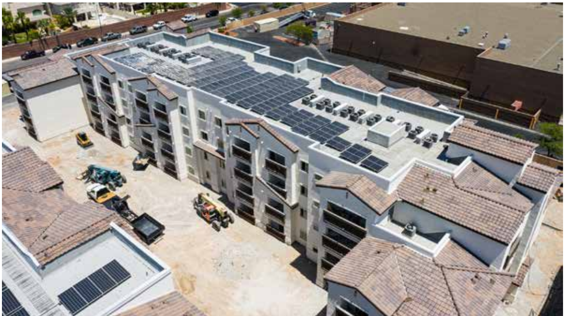
Photo (Above): Flamingo Pines Senior Apartments - 66 apartment units of low income senior housing. Las Vegas, NV. (Source: NV Energy/Clearesult).
