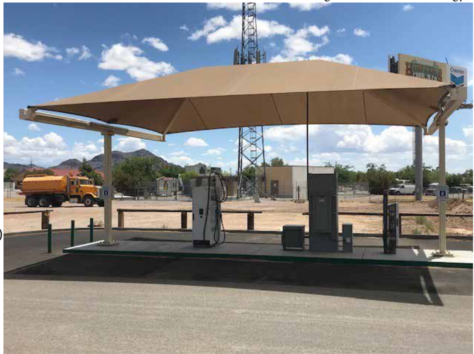
Photo (Above): Amargosa Valley NEH charging station at the NDOT rest stop in Lathrop Wells, NV. (Source: Valley Electric Association).
